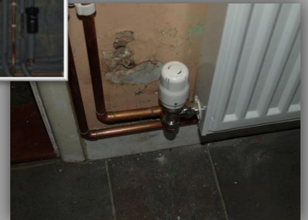
AFTER: Brand new radiators including, new pipework and thermostatic radiator vales.
